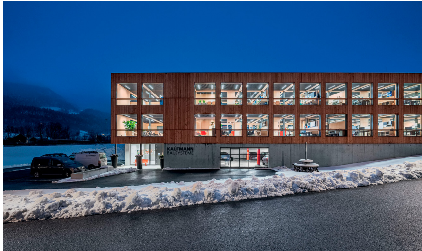
The 54-metre-long new building for Kaufmann Bausysteme, which extends over two storeys and consists of a total of 32 individual modules, was completed in record time: just 18 months from the first draft to moving in, thanks to the modular construction method.
